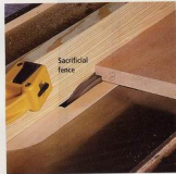
Cut the tongues on the edges of the side panels using a dado stack in your table saw (plus a sacrificial fence). You also could use a rabbeting bit in your router table.
